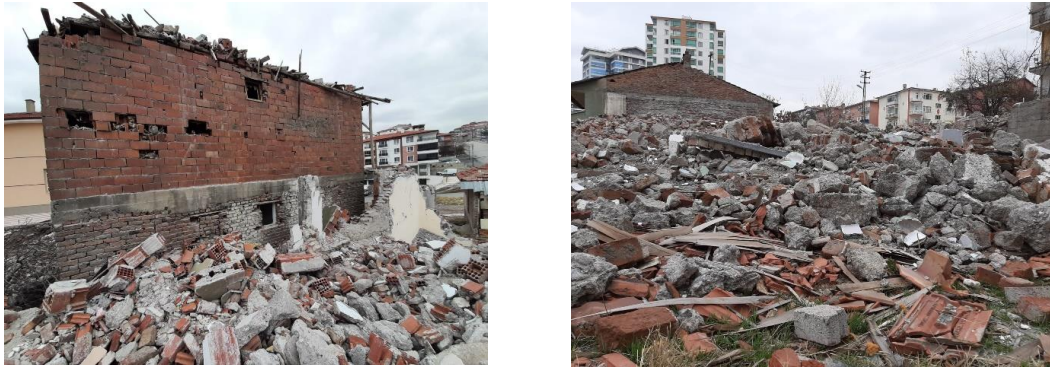
Figure 1. Demolition site in Ankara/Turkey
