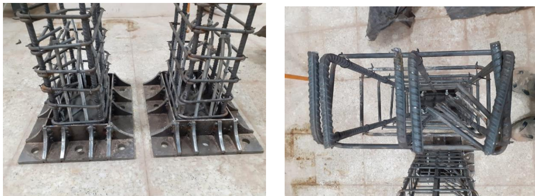
Figure 3-38 Details of connection point of demountable column 4
