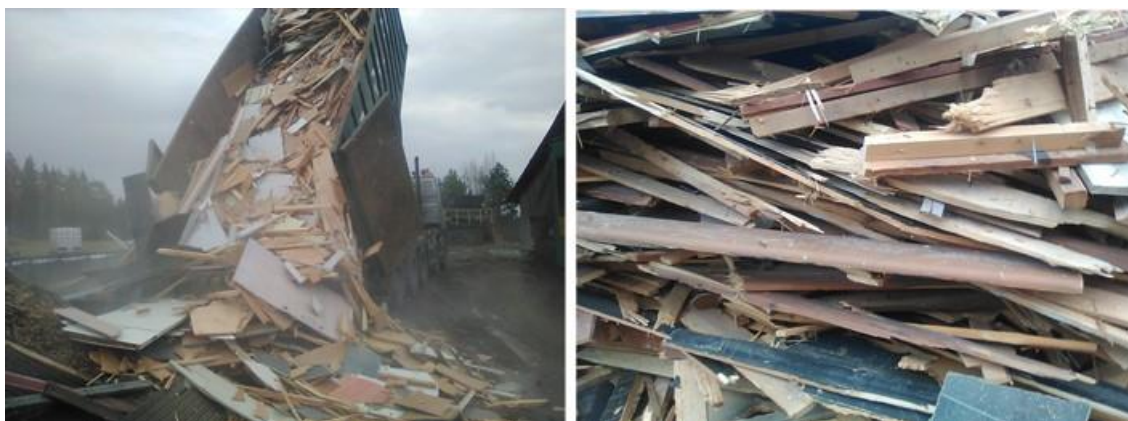
Figure 7-4. At left Raw materials from Purkupiha, at right mixed C&D wood waste
