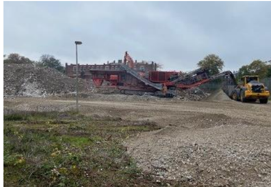
Figure 21. Crushing the EOL concrete with a mobile crusher
