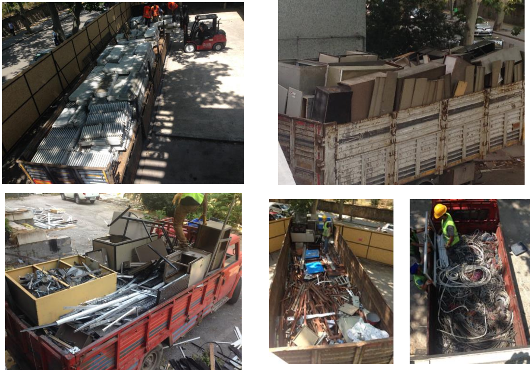
Figure 47. Transportation of all materials obtained from building
