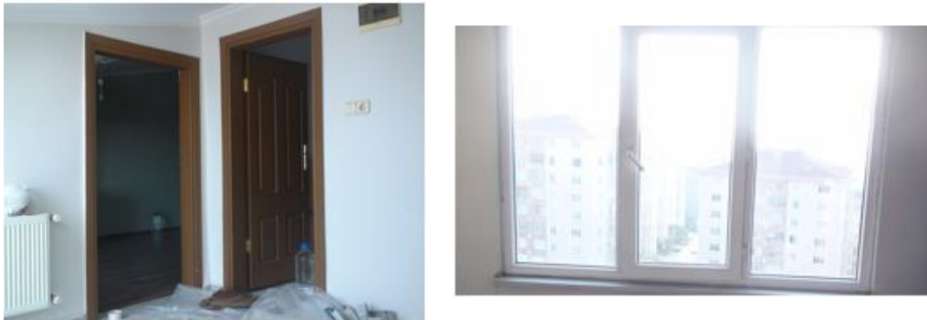
Figure 39. Interior visuals of the building to be demolished
