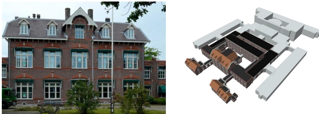
Figure 2. The Eikenstein detention center in Zeist, Netherlands. The grey area is the non-monumental part that is deconstructed (within the scope of ICEBERG).
