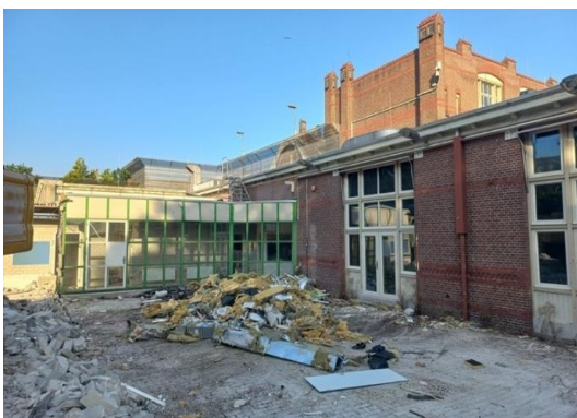
Figure 9. Collection of insulation materials (photographed by Frank Rens and Bente Kamp, GBN)
