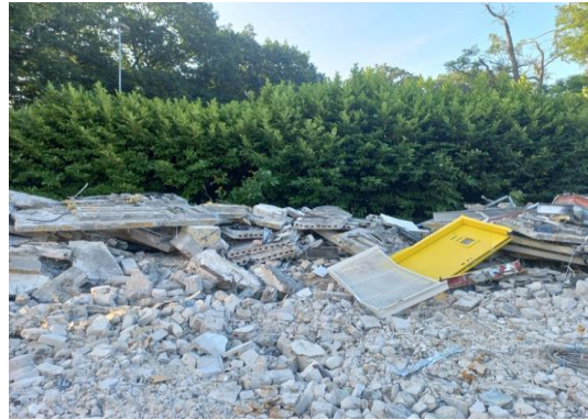
Figure 16. Mixed waste before separation on site (photographed by Frank Rens and Bente Kamp, GBN)
