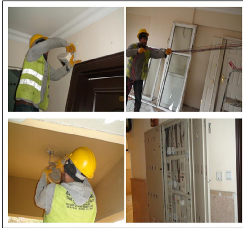
Figure 43. The cables and other components removed without damage before demolition
