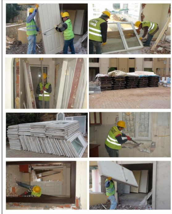
Figure 42. The dismantling of elements such as doors and windows
