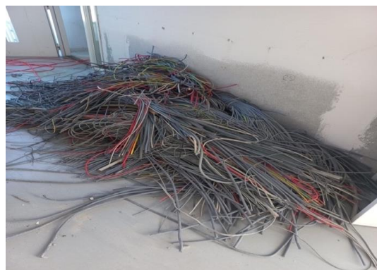
Figure 10. Collection of cables (photographed by Frank Rens and Bente Kamp, GBN)
