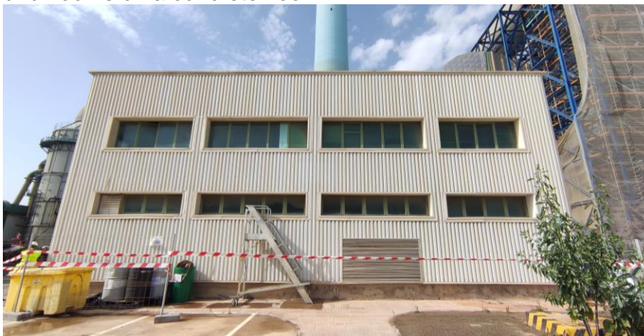
Figure 72. Main facade of the electrical building which was demolished.
