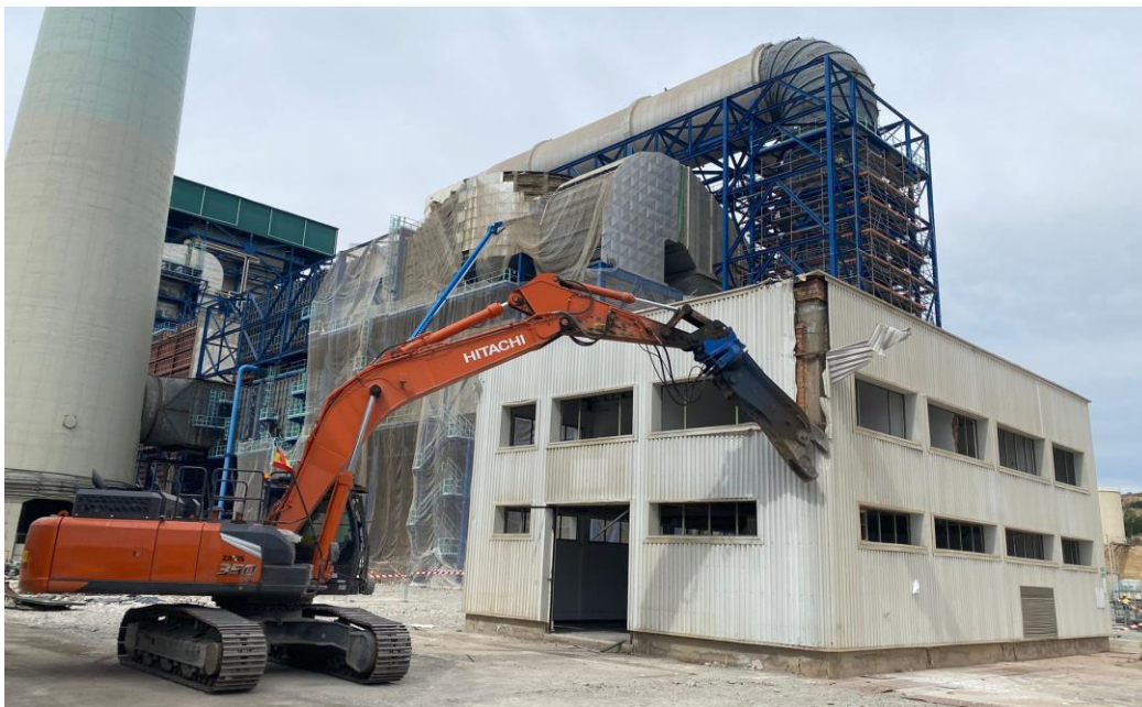
Figure 84. Dismantling of the covering of the building.
