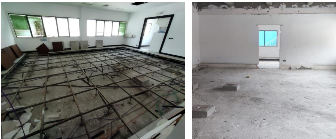
Figure 76. Raised flooring dismantling process.
