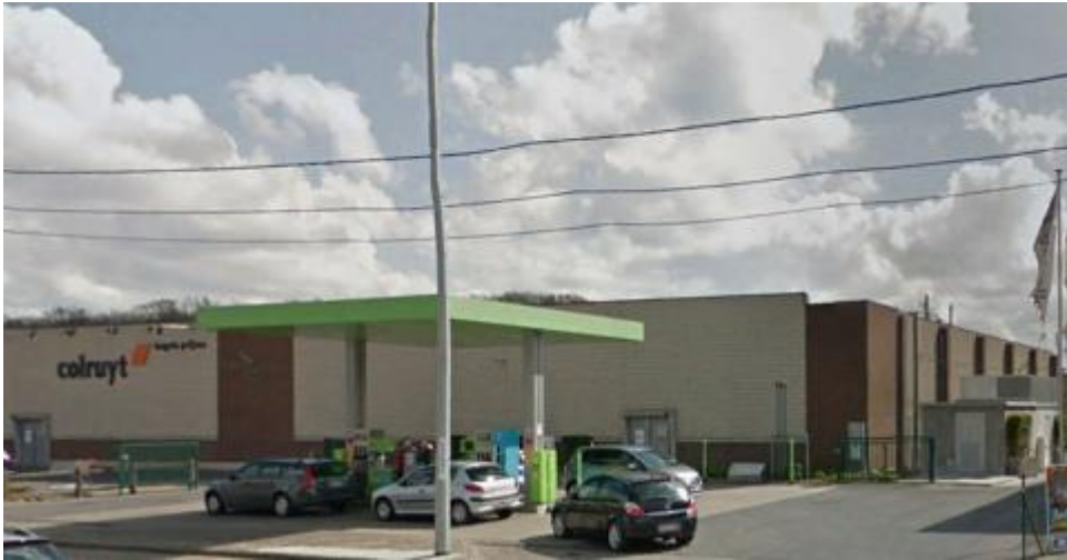
Figure 49. The demolition case study (the petrol station in the front is not part of the demolition works) (address: Gampelaerreedreef 1, 9800 Deinze, Belgium).
