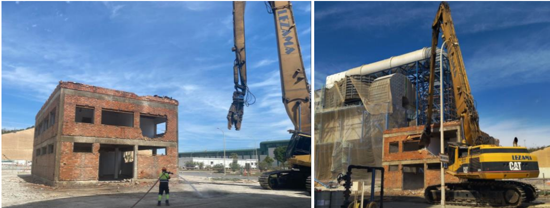
Figure 85. Machinery demolition of the structure.
