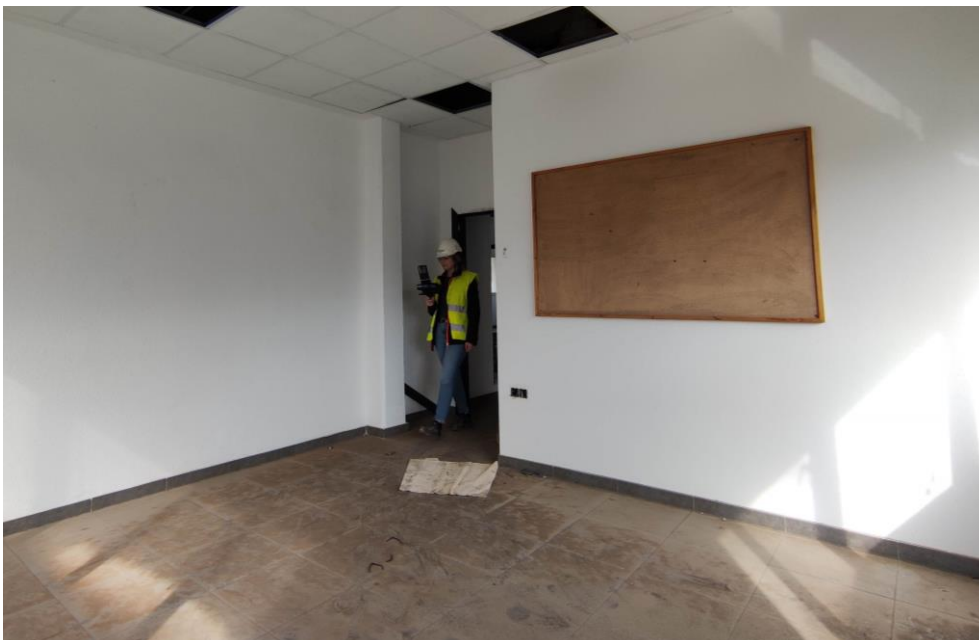
Figure 74. Scanning process by TECN.
