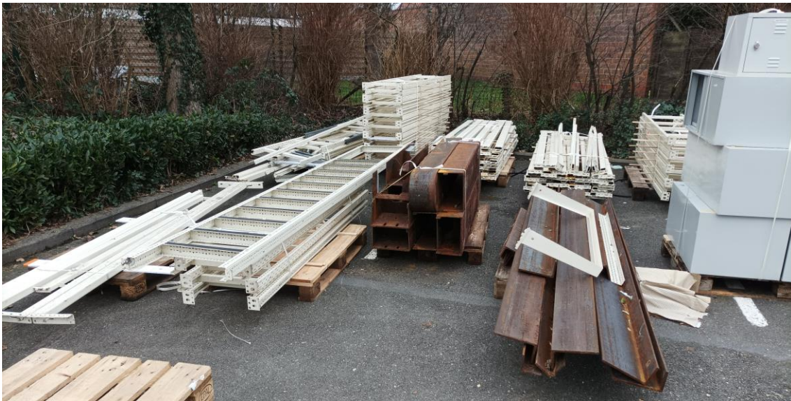
Figure 52. Some elements that were selectively removed for reuse.
