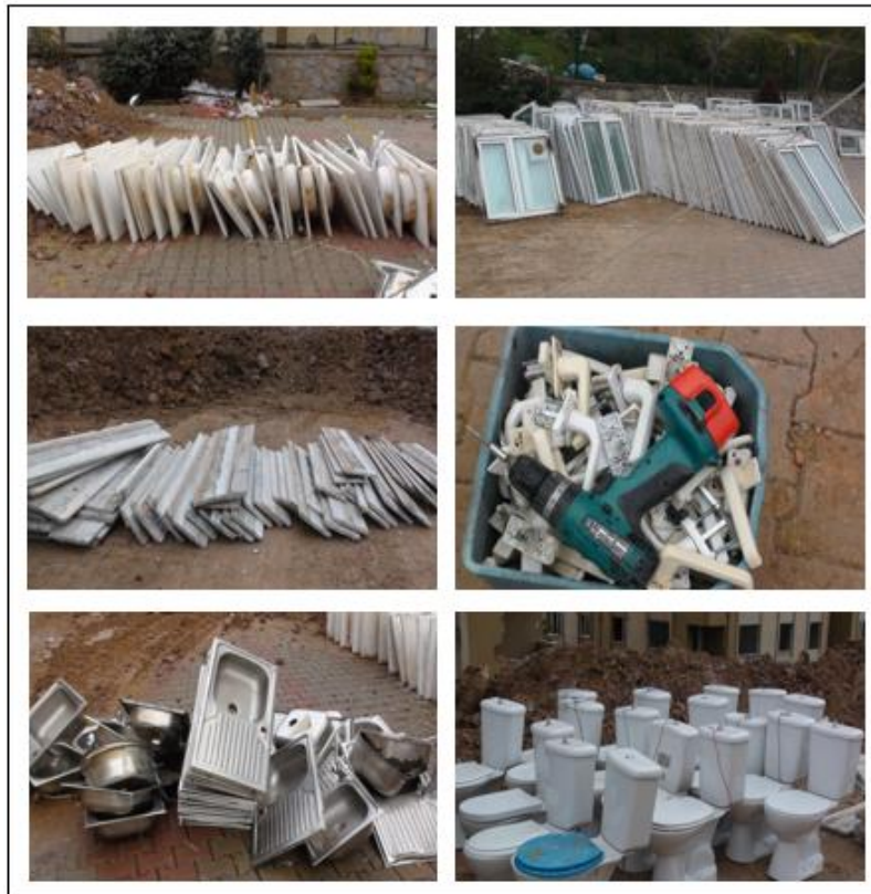
Figure 45. The steel, wooden, PVC doors, and PVC windows removed from the demolished building
