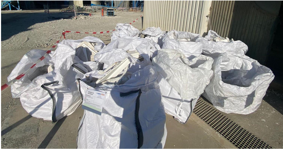
Figure 83. Waste streams segregated during the internal demolition process.
